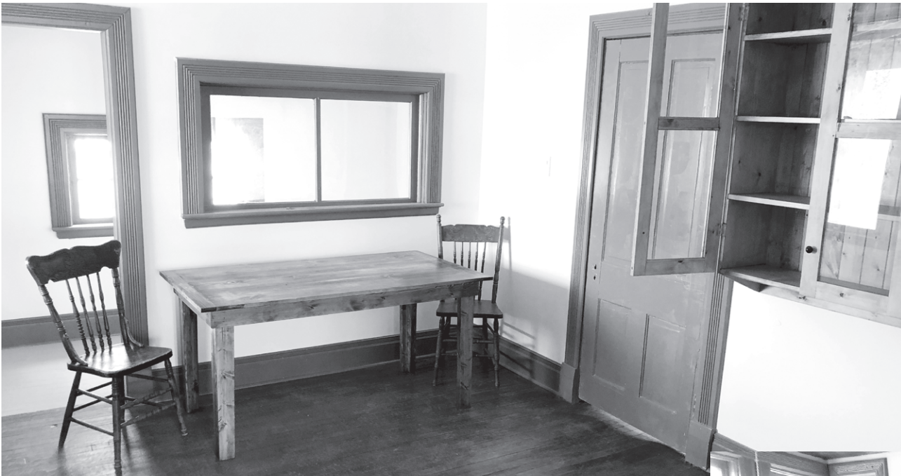
The La Riviere CPR Station was moved from Archibald Museum to the railway track at Manitou. Many hours of work has gone into restoring the old building. To the left is the restored kitchen in the north side leanto.
